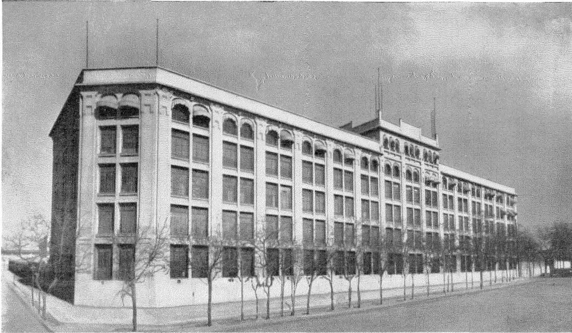
Fig. 9—The Madrid factory of Standard Electrica, S. A., one of the two I.T.&T. plants in Spain.
